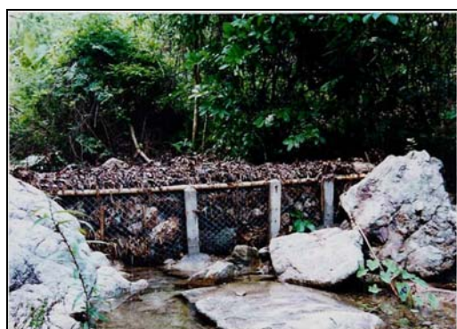
Figure 1. Temporary check dam construction
