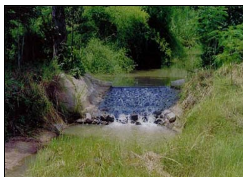
Figure 2. Semi - permanent check dams construction
