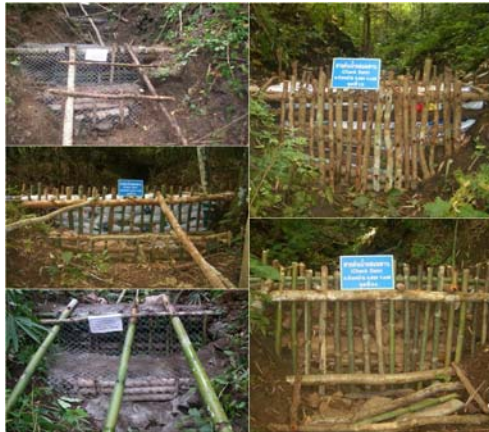
Figure 8. Example of check dam construction at Doiluang Wildlife Sanctuary, Thailand
