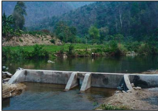
Figure 3. Permanent check dams construction
